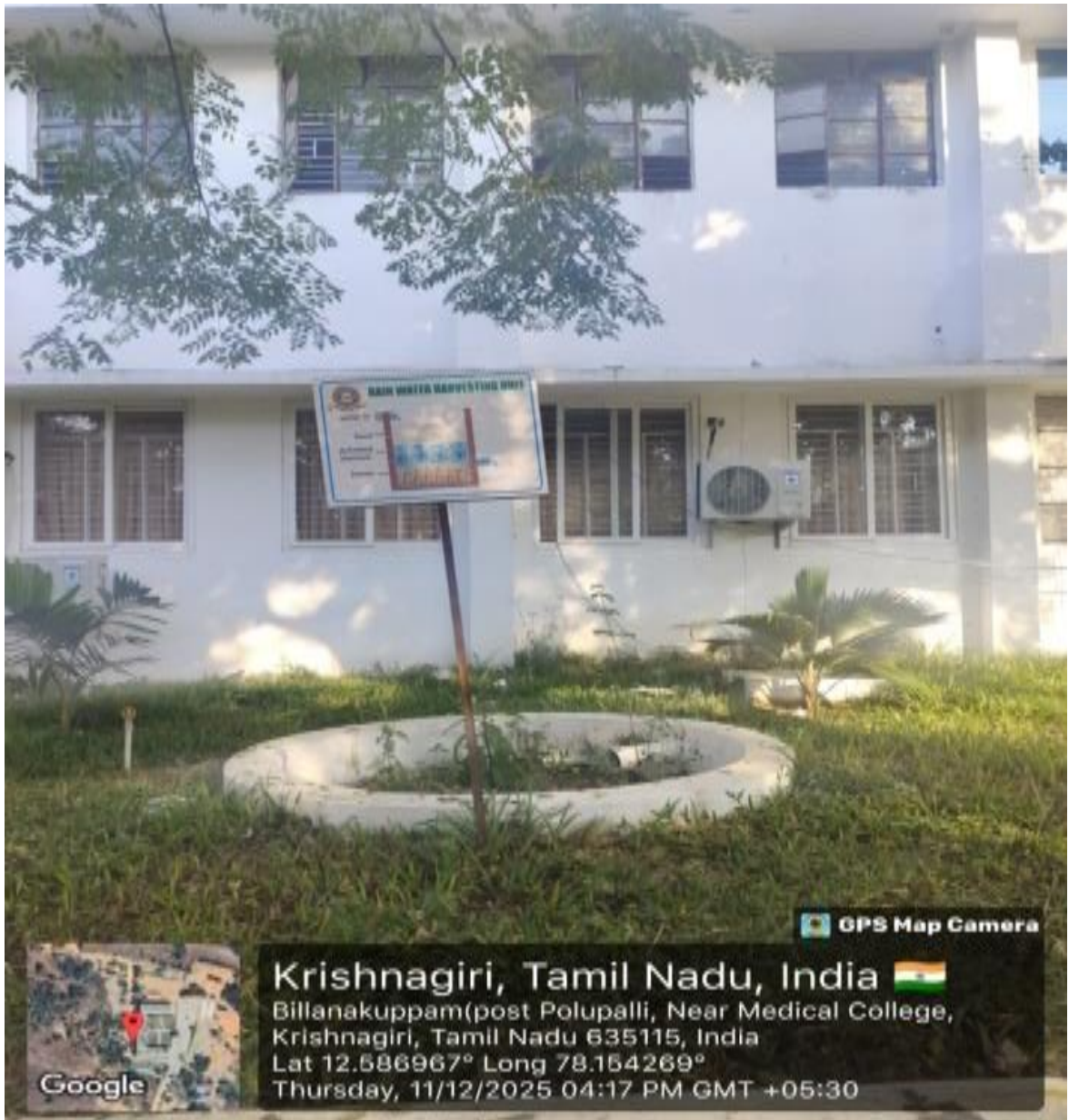
RAIN WATER HARVESTING TANK IN C BLOCK
